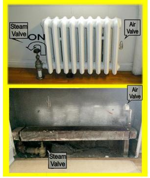
When valve is turned counter-clockwise all the way, the valve is <u>**ON**</u> and the radiator will <u>**HEAT**</u> when the steam is available.
